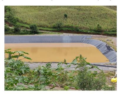
The Temporary Receiver and her team took immediate action to prevent the dam from overflowing, including the pumping of water out of the tailings dam to avoid further damage. The
